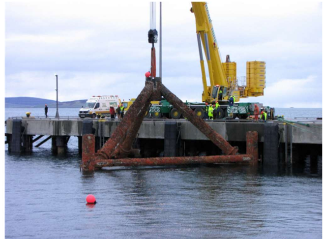
Lift 2 with central vertical member and lower horizontal members removed
