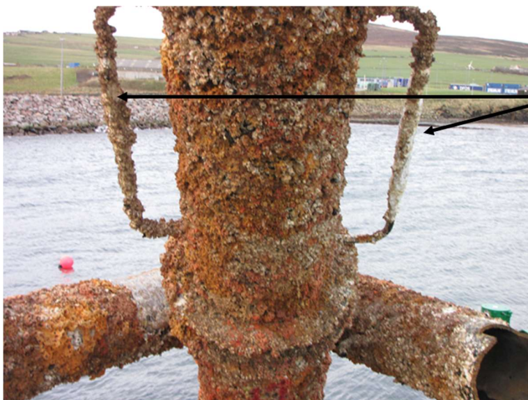
Figure 28 - condition of anodes after 11 years
