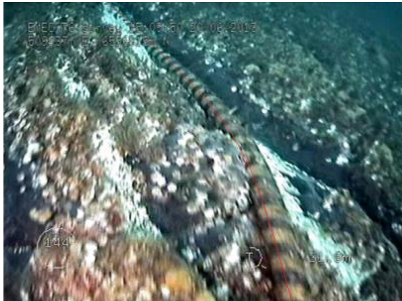
Figure 12: Rock contact with cable T7
