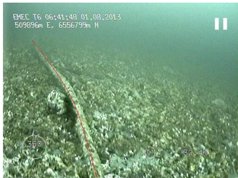
Figure 10: Rock contact with cable W2
