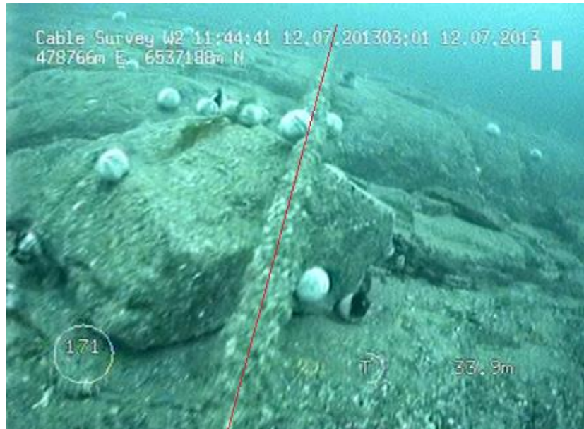
Figure 10: Rock contact with cable W2
