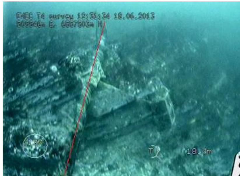
Figure 13: Interaction of fishing creel with EMEC cable T4
