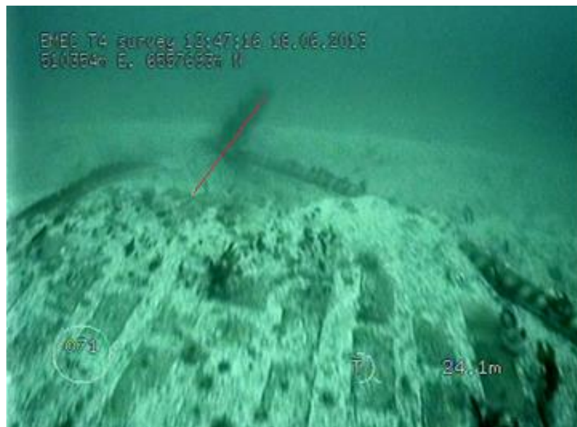
Figure 14: Mattress crossing T4 with T6 (cables in contact)
